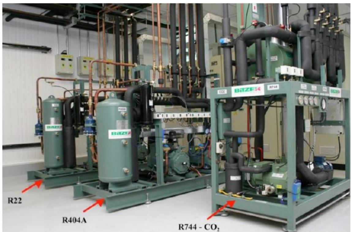
Figure 3.11 R22, R404A and CO 2 /R404A refrigeration systems trailed by BITZER for supermarket application
