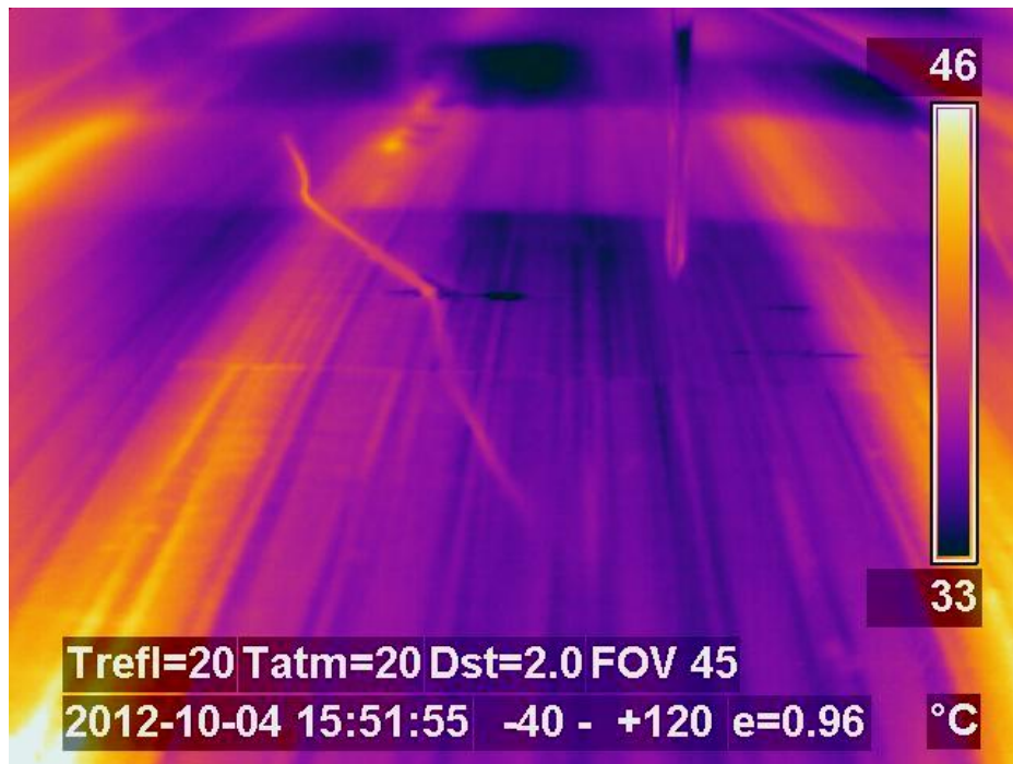
Figure 7.6 Thermal imaging capture
